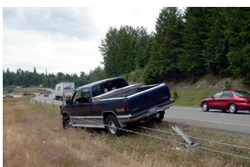
Example of cable median barrier benefits (left) [FHWA].
